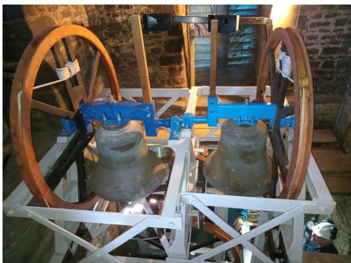
The Treble bell on the right with new Headstock with Twiddle pins fitted
